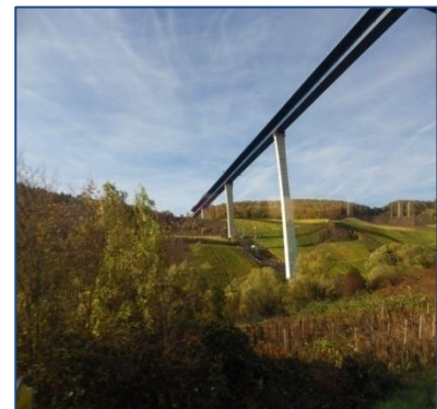
The view of the bridge from below at Rachtig
